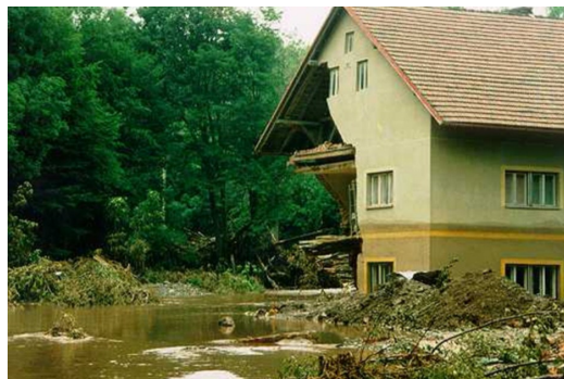
The damage was tremendous © MRBA
