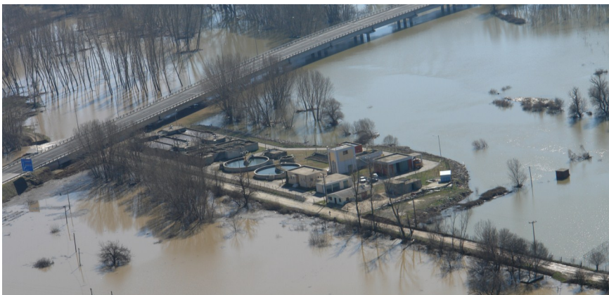
Area of Didymoteicho Wastewater Treatment Plant (taken on 19 February 2010). ©George Tsesmelis, Alexandroupolis Aero Club.
