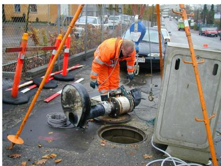
Preparation of sampling and flow measurements in Gladsaxe
