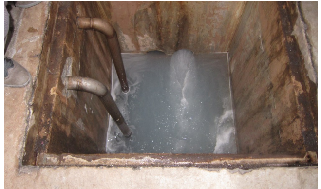
Discharge water from the boiler and continuous batch washer that has recycling potential. © DHI
