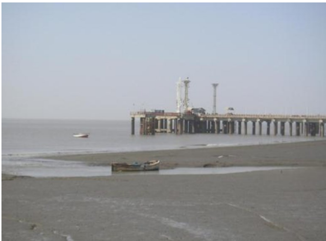
Existing RDMT Jetty head
