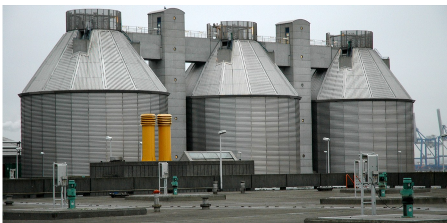
Anaerobic sludge digestion tanks at Lynetten Wastewater Treatment Plant.
