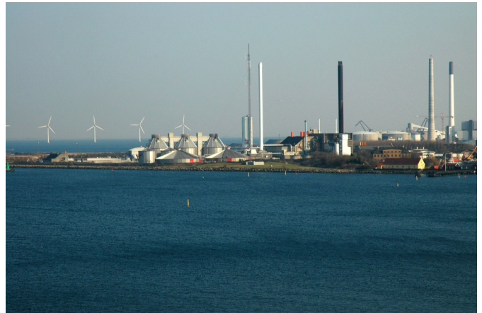
Lynetten Wastewater Treatment Plant treats wastewater from Copenhagen, Denmark.
