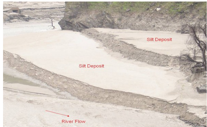
Typical sedimentation pattern in a ROR scheme.
