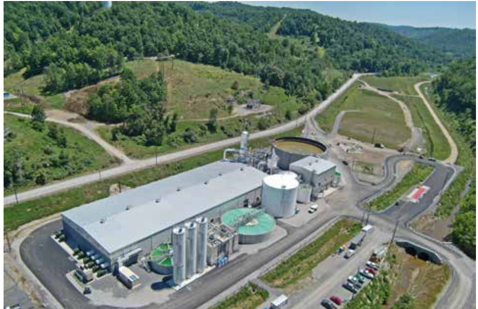
A Veolia Zero Liquid Waste facility
