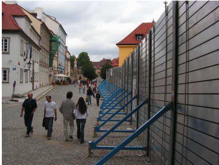
Fig. 2 One of the selected critical places with high mobile barriers – Na Kampě
