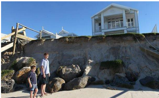
Figure 1 Example of erosion at Palm Beach
