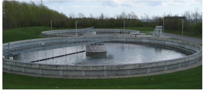
Model of a secondary settling tank requires advance modeling like viscous effects (plastic behaviors), hindered settling, in order to captures the formation of a sludge blanket
