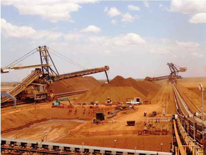
Stacker, reclaimer and conveyor system (Source: FMG). © FMG
