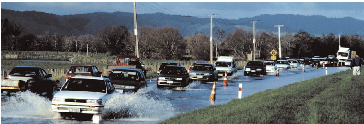
Figure 4 Cars on State Highway 1 during the operation of the Rangiriri spillway
