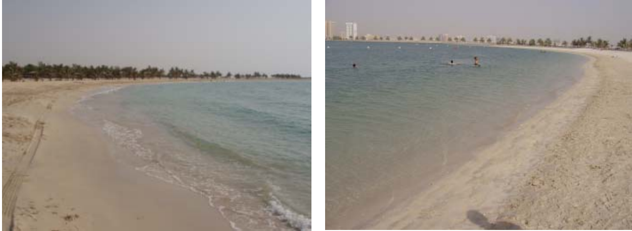
Figure 3. Mamzar Beach in Dubai. Left: good quality exposed artificial beach at the Mamzar Sea Beach. Right: moderately good quality protected artificial beach at the Mamzar Lagoon Beach. The fill sand is in both cases medium well sorted with no content of fines or coarse material.
