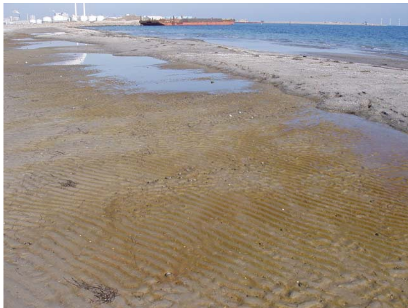
Figure 13. Development of beach bar and beach lagoon with algae growth on the shallow shoreface at Amager Beach Park during the construction process.
