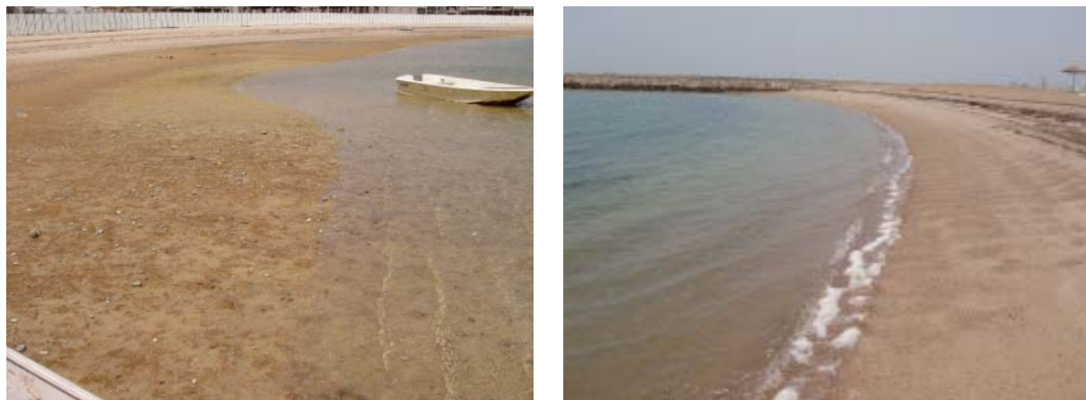
Figure 2. Artificial beaches north of Doha, Qatar. Left: a very protected location. Beach material is fine graded sand with content of both fines and coarse material, the shallow shoreface is suffering from siltation of fines. The beach is swampy and wet with greenish algae areas and the beach is occupied by crab pellets and scattered shingle, all in all an unattractive beach. Right: same location, but a little more exposed and the beach has been built of medium well sorted sand. This beach has a much nicer appearance; however, it has more the character of a sand slope than of a beach. It suffers from siltation of fines and the shoreface is muddy at water depths greater than approx 0.3 m.
